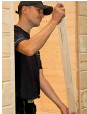
Windows and doors are mounted on guide rails to increase stability and tightness of fit
