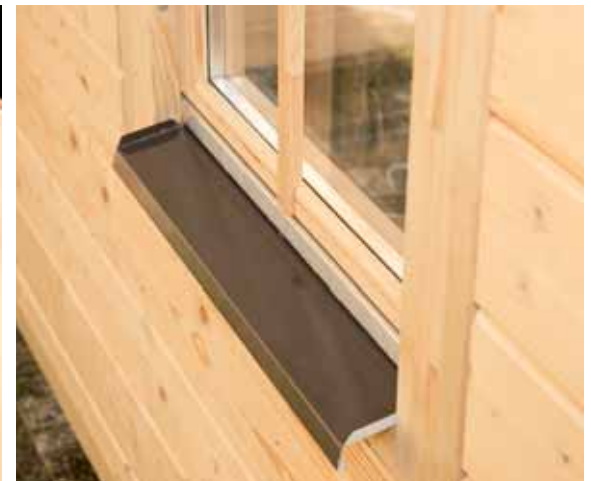
Window frame in glued laminated timber with concealed frames, windows with insulated glass and aluminium nose drop
